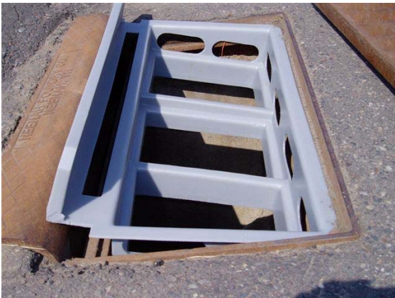
Remove grate and set frame on top of casting
