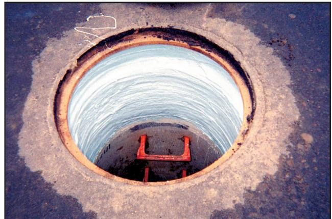
An inexpensive and permanent method of sealing the grade adjustment ring area and joint sections in a manhole or catch basin from the inside of the structure. This state-of-the-art urethane material is packaged in a kit that is easily applied by SSI certified installers.
