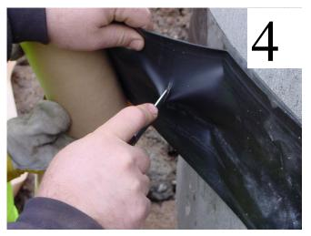
4. Cut excess material using a utility knife. Using a rubber mallet or hand held roller, firmly flatten the Gator Wrap® 360 degrees around joint.
