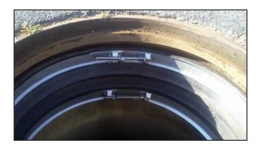
The **S.S.I. INTERNAL UNI-BAND** can be used on existing and new construction manholes or catch basins. A clean surface is necessary but no special tools are required for installation.
