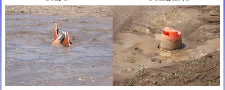
The Sediment Control Barrier utilizes a filtration process that prevents sediment and construction debris from entering the sewer system after a rainfall. It also allows water to percolate through perforations to reduce construction downtime and costs. The Sediment Control Barrier is manufactured by Royal Environmental Systems
